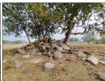
Plate III Dilapidated temple, Shasandih
