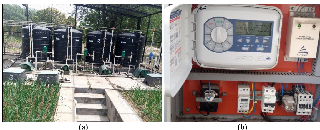
Fig 3: Components of the automatic irrigation system (a) and controller box (b)
